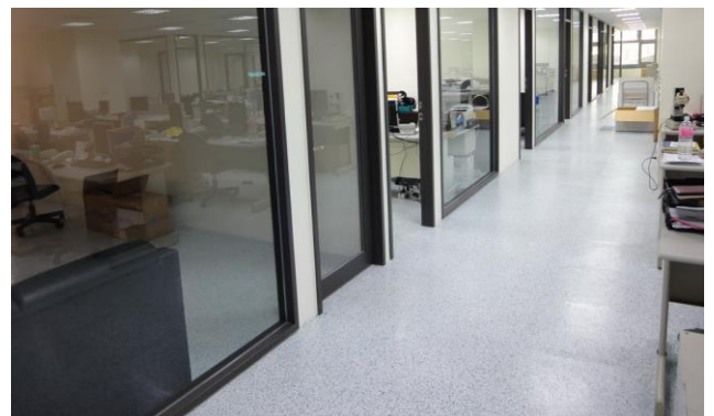
office renovation project, top-finish by vinyl tiles
