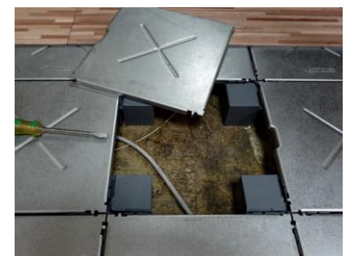
lift Top-Panel by screw driver
